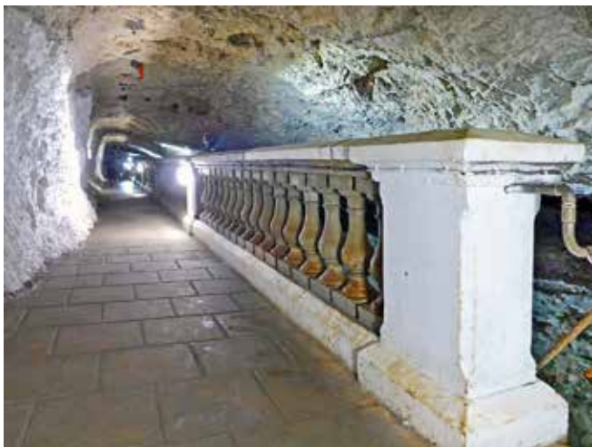
Reservoir No.8 (1936): the reservoir chamber is to the right, below the level of the balustrade
